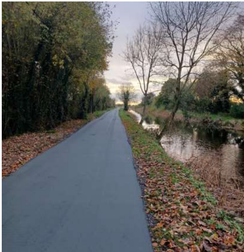
Fig1 – BallyKelly to Hugh Bridge looking South. Section completed Dec 2022
