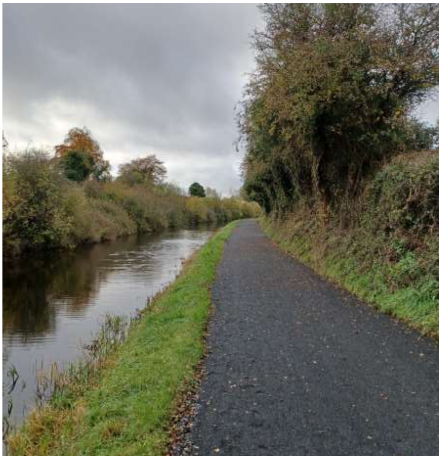
Fig 3 – CH25000 looking south. – Completed Blueway.
