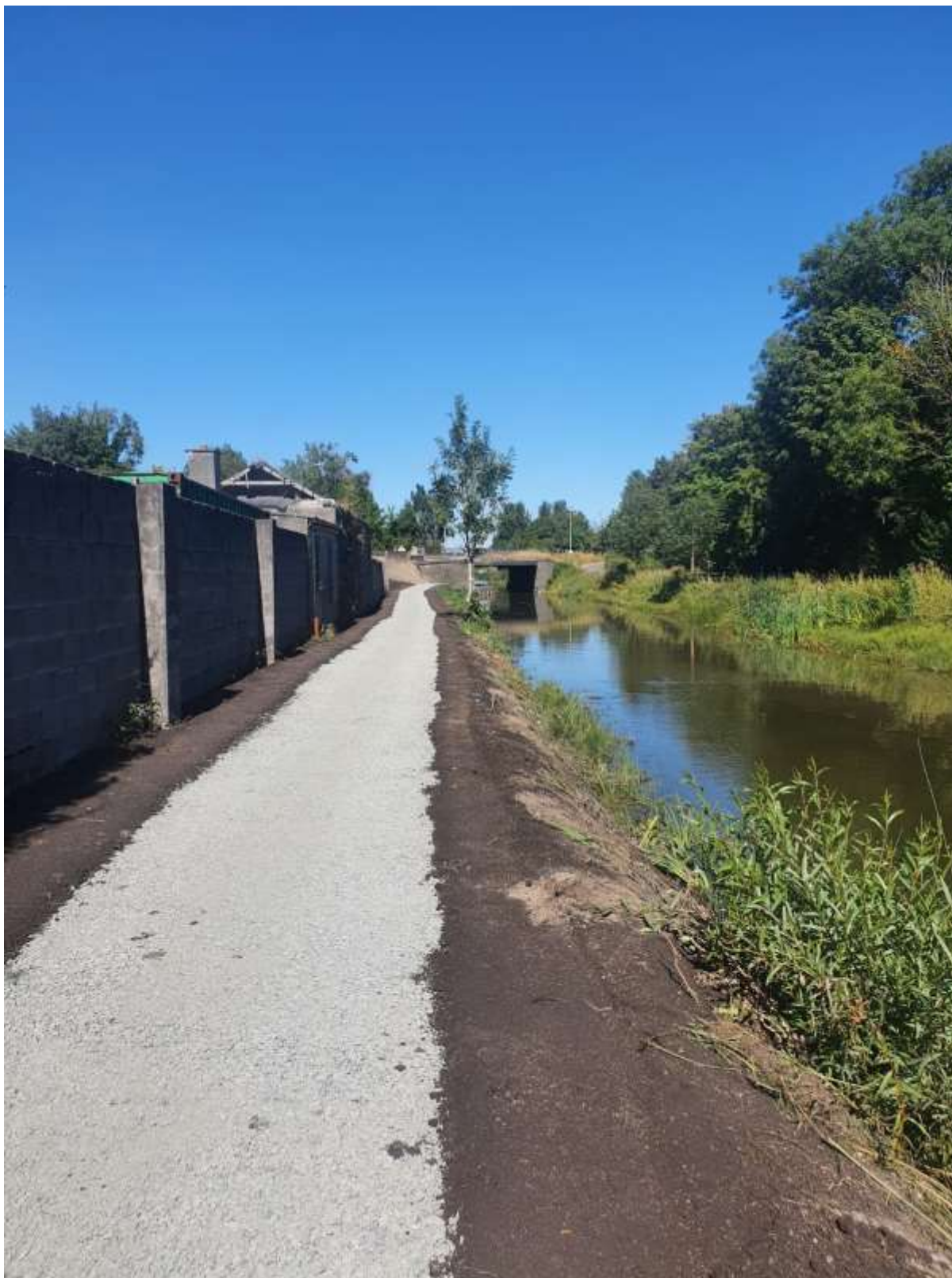
Fig 2 – CH24340m, Looking North. Clogheen Bridge
